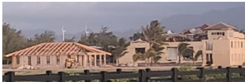
The historic buildings at Marconi Point being renovated a few years ago.
