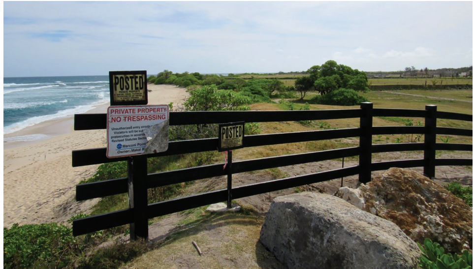
A 2022 photo of a portion of the unauthorized fence at Marconi Point in the Conservation District.
