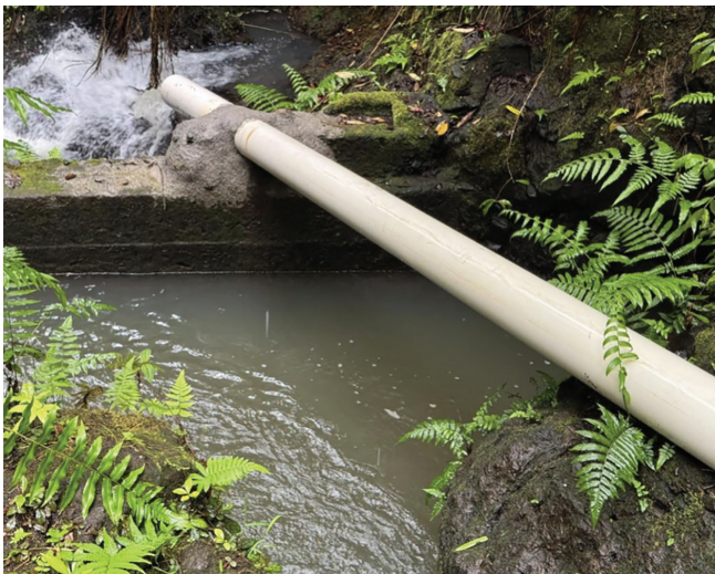
An enlarged pipe in the Lowrie Ditch at Hanawana Stream (left) is one of the completed modifications. An open sluice gate on O'opuola Stream is one of the voluntary, temporary measures that have been implemented pending permit approvals for permanent modifications (right).
