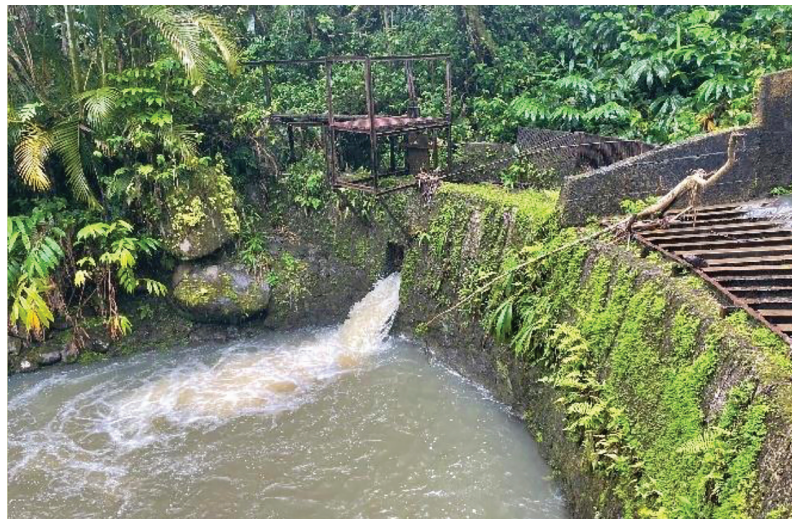
An enlarged pipe in the Lowrie Ditch at Hanawana Stream (left) is one of the completed modifications. An open sluice gate on O'opuola Stream is one of the voluntary, temporary measures that have been implemented pending permit approvals for permanent modifications (right).
