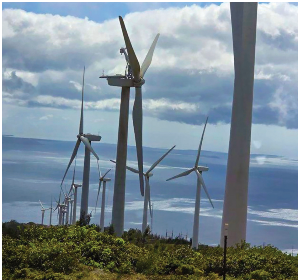
Kaheawa wind farm. CREDIT: DLNR.
