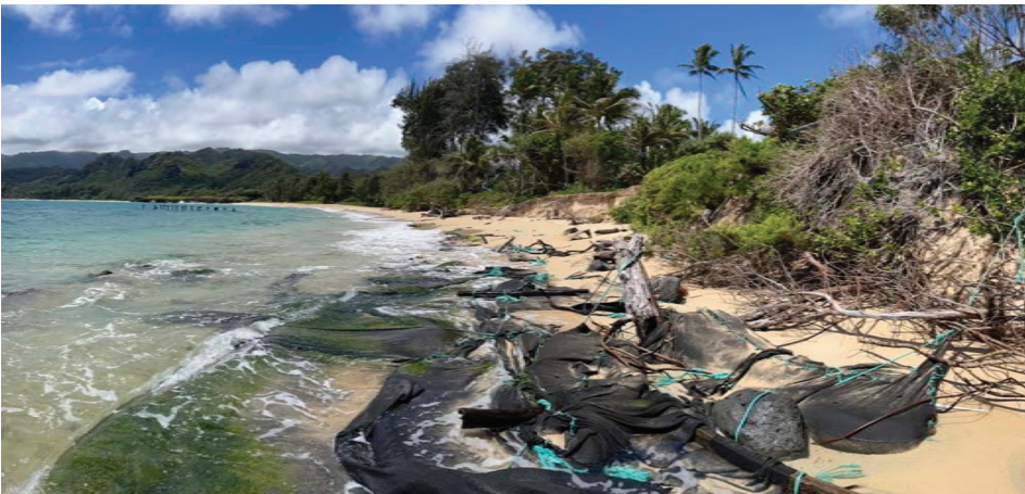
A photo taken by Office of Conservation and Coastal Lands last year of debris from the Greigs' emergency erosion control structure in Lā'ie installed in 2017. CREDIT: OCCL.
