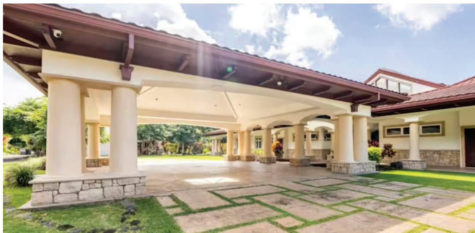
The exterior of Eisert's vacation rental property. CREDIT: VRBO.COM.
