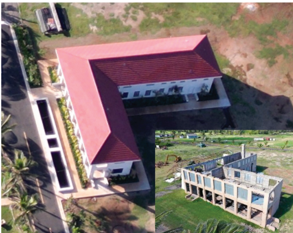
The hotel as it stands today. The inset photo shows how it looked in 2021.
