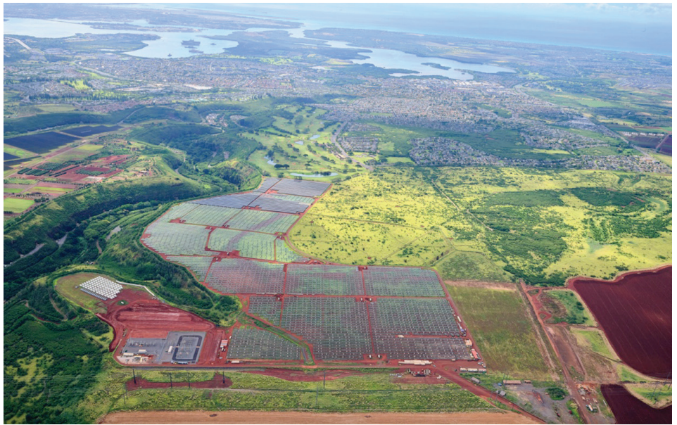
View of the Ho'ohana Solar installation, looking toward Pearl Harbor. CREDIT: HO'OHANA SOLAR.
