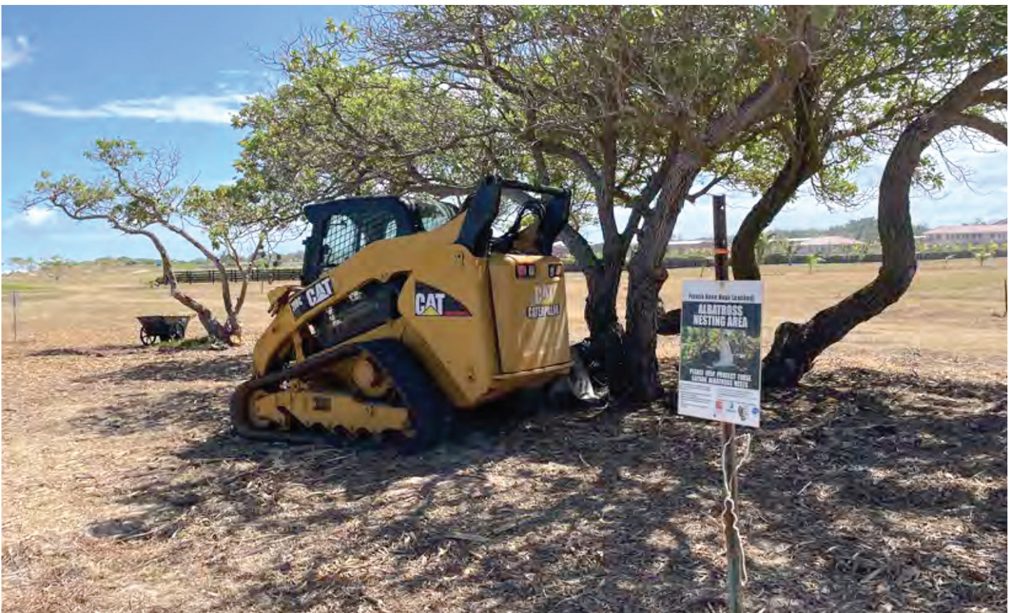
Heavy earth-moving equipment is parked next to a posted notice that this is an albatross nesting area. CREDIT: DLNR.
