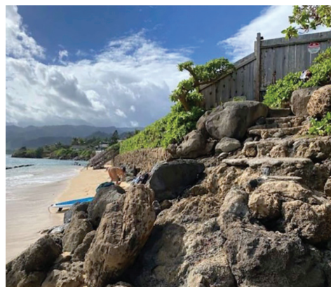
The revetment and stairs at Lā'ie for which the Land Board recently approved a 25-year easement.
