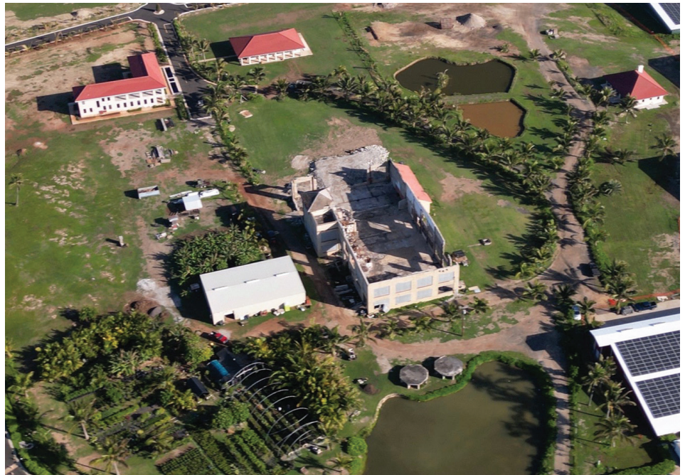
The historic buildings at Marconi, one of which was recently damaged during renovation. CREDIT: PETER FOWLER/ENDURE FILMS.
