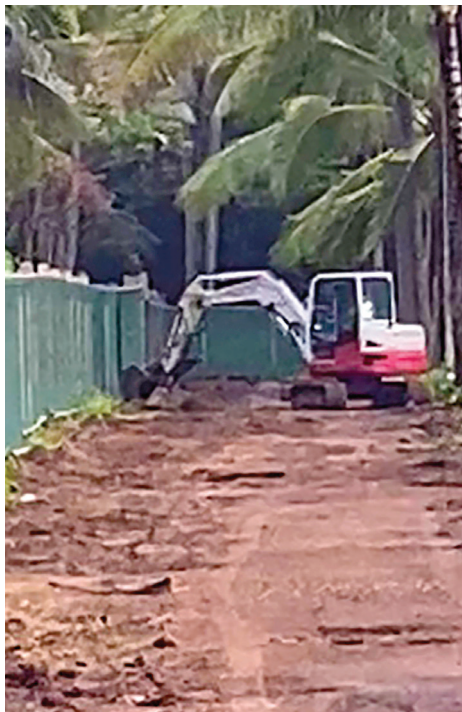
A lone backhoe operator digs a hole near the coconut grove area of the former Coco Palms Resort site.
