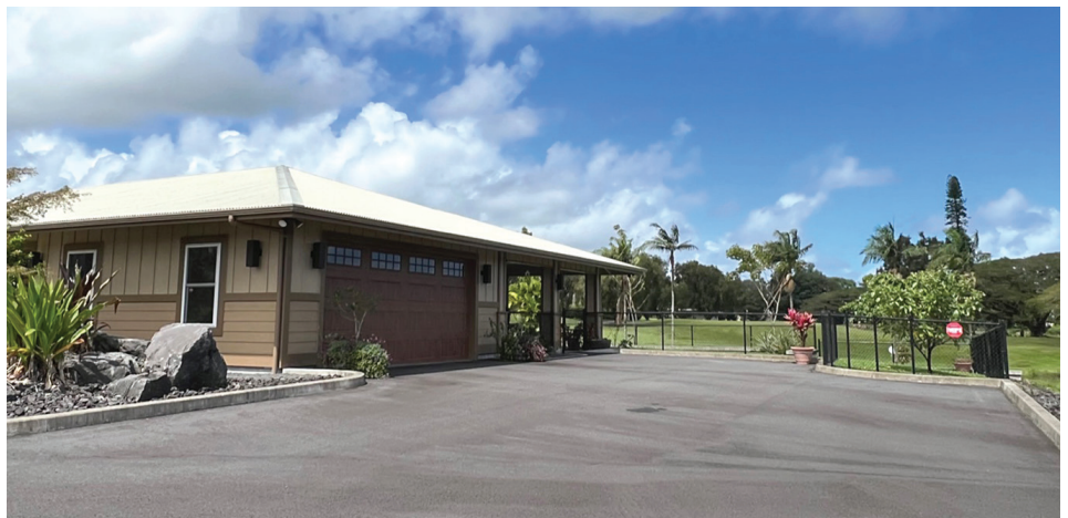
Many houses in the Waiiaka Fairways subdivision back up against the Hilo Municipal Golf Course.
