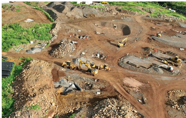
An aerial view of the Kauanoe o Koloa luxury condominium development in December 2022. Blasting had been completed, pipes were being laid, and building pads prepared. CREDIT: KAUANOE O KOLOA
