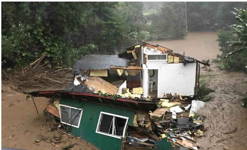
Flood damage from an April 2018 severe rain event in north Kaua'i. “This climate change-induced ‘rain bomb’ ... cut off road-based access into and out of Kalā’s community for several weeks,” the youth plaintiffs’ complaint states. CREDIT: UH SOEST
