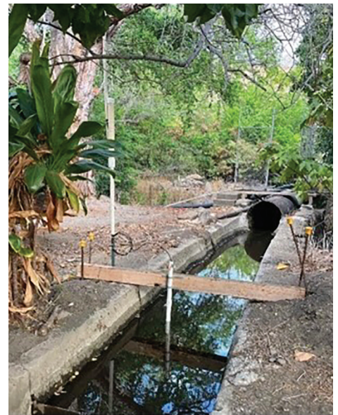
A new data logger to measure Olowalu Water Company's diversion. CREDIT: CWRM
