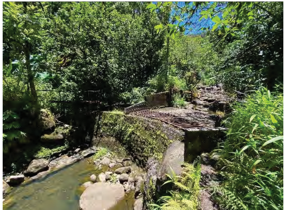
Spreckels Ditch intake at 'O'opuola Stream where staff recommends placing a plate to improve connectivity. CREDIT: CWRM
