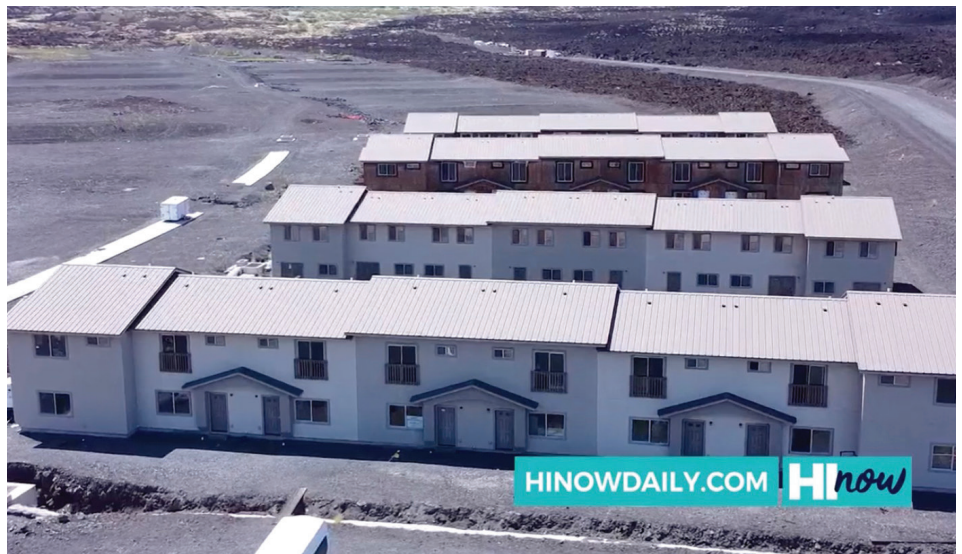
These affordable units built by 'Aina Le'a more than a decade ago are still not ready for sale.
