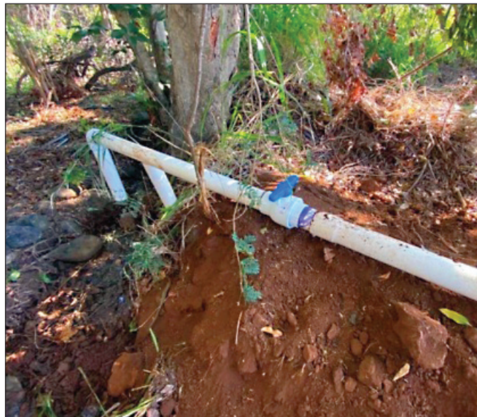
The 4" line into the South Waikapū kuleana 'auwai.
