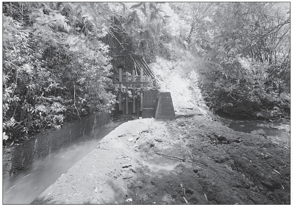
East Maui Irrigation supply aqueduct going into tunnel, in vicinity of Na'ili'ihiha'ele Bridge - Hana Belt Road, Between Haiku and Kaipahulu.
